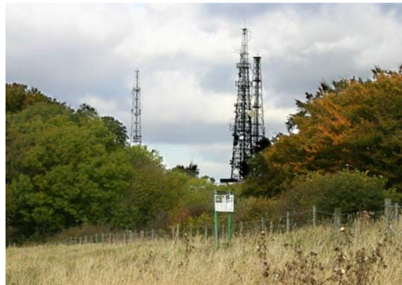
Telecommunication masts above Masts Field
