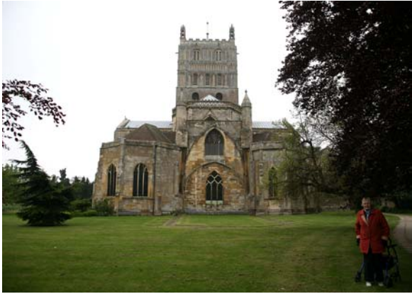
N elevation of Tewkesbury Abbey
