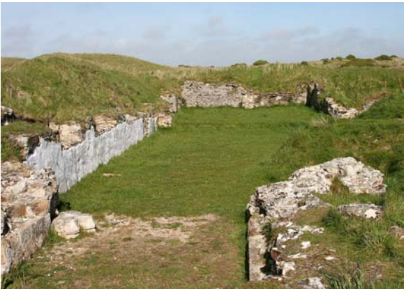
Foundations of the second St Piran's church on Penhale Sands. It was abandoned in 1804
